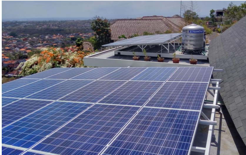
Two Array's of 20 solar panels each. Total capacity 10,000 Wp.
