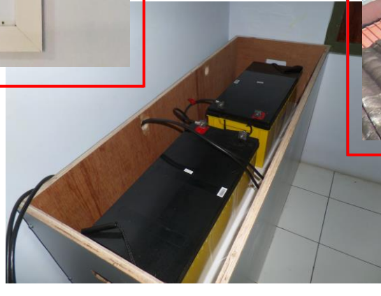
Battery Bank Capacity 9.6 kWh.
